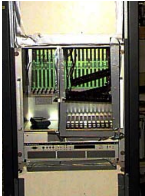
Figure 1 Front view of the rack test. The VME crate is shown. The heat exchanger is hidden in this picture. Several resistors are shown in the 9U section of the crate.
