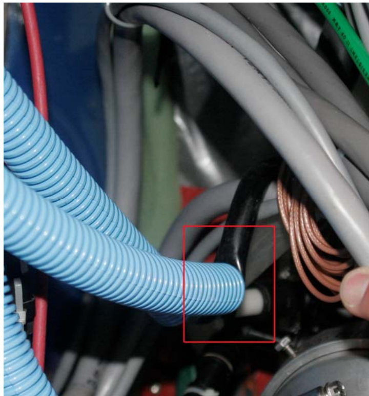
Figure 10: The red box highlights a kinked cooling hose that was discovered during the removal and disassembly of the SSD in August, 2007. Ideally, the blue corrugated hose should have protected the black vacuum line ... but didn't in this case.
