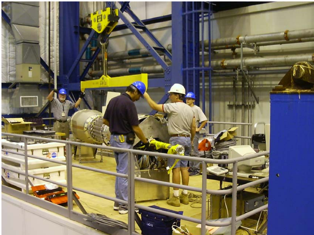
Fig.14: lifting operation of the cone with it dedicated lifting beam.
